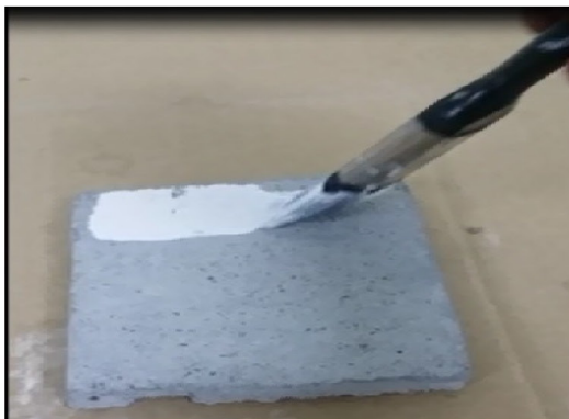
Applying paint on SealPov treated surface
